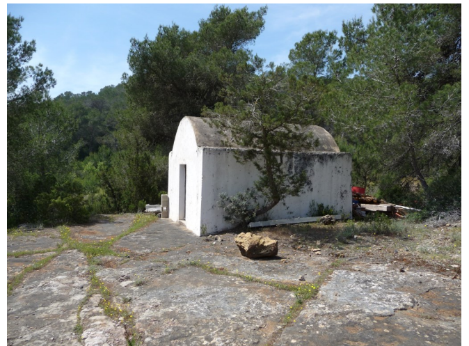
Diverse infrastructures of the San Jorge pit. Explosives magazine of the mines of Ibiza
